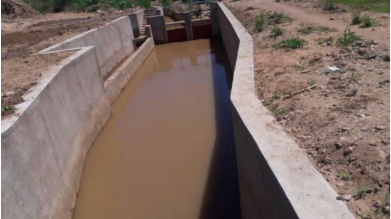
Figure 6. Magozi reconstructed water intake.
